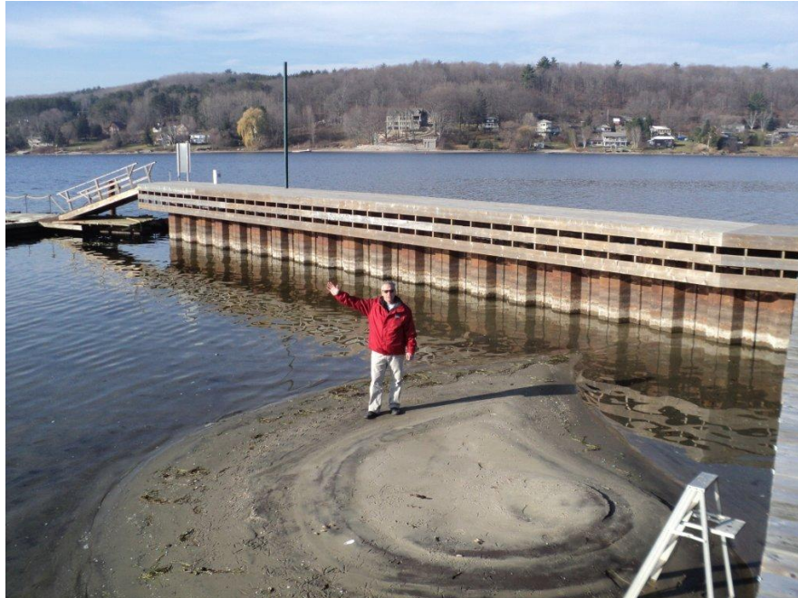
Assistant Marina Manager at Bay Moorings, standing where part of their dredging efforts are taking place this winter.
